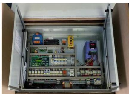
Of particular interest for this project is the Optidrive Elevator's renowned ability to deliver smooth carriage through its use of no less than five independent S-shaped acceleration ramps. Along with a dedicated motor holding brake control algorithm, this allows fine tuning of the system by installers. Then there are Optidrive Elevator's compact external dimensions and factory parameter settings that are well-suited to fast, easy installation and setup of simple elevator applications.
